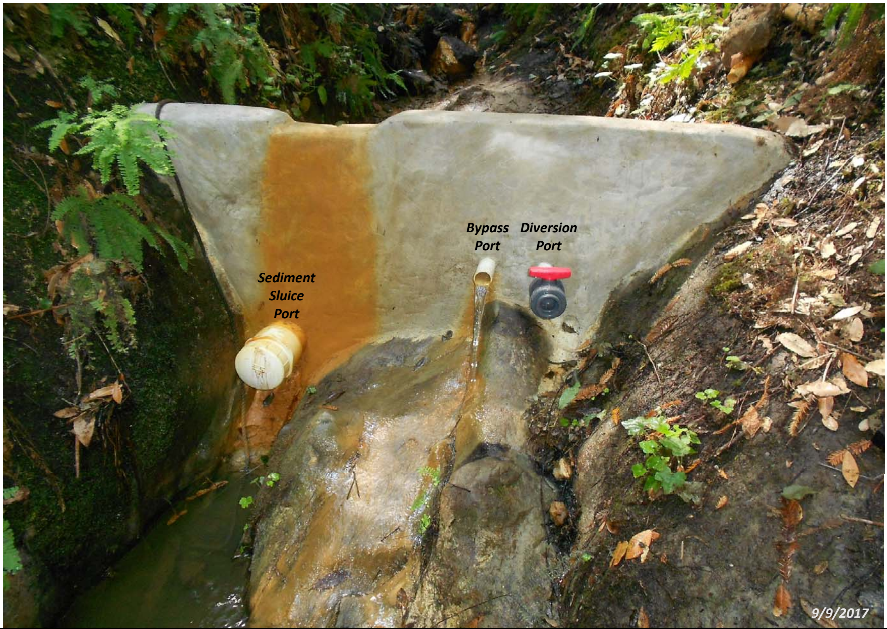
Figure 6. Improved diversion structure on Piney Creek, Redwood Glen, San Mateo County, CA. The diversion structure was rehabilitated during 2017 to remove sediment and debris, and to restore its full functionality. It now includes a functioning bypass port and diversion port with the same diameter and set at the same elevation. If both ports are completely open, then the flow is passively split in half.
