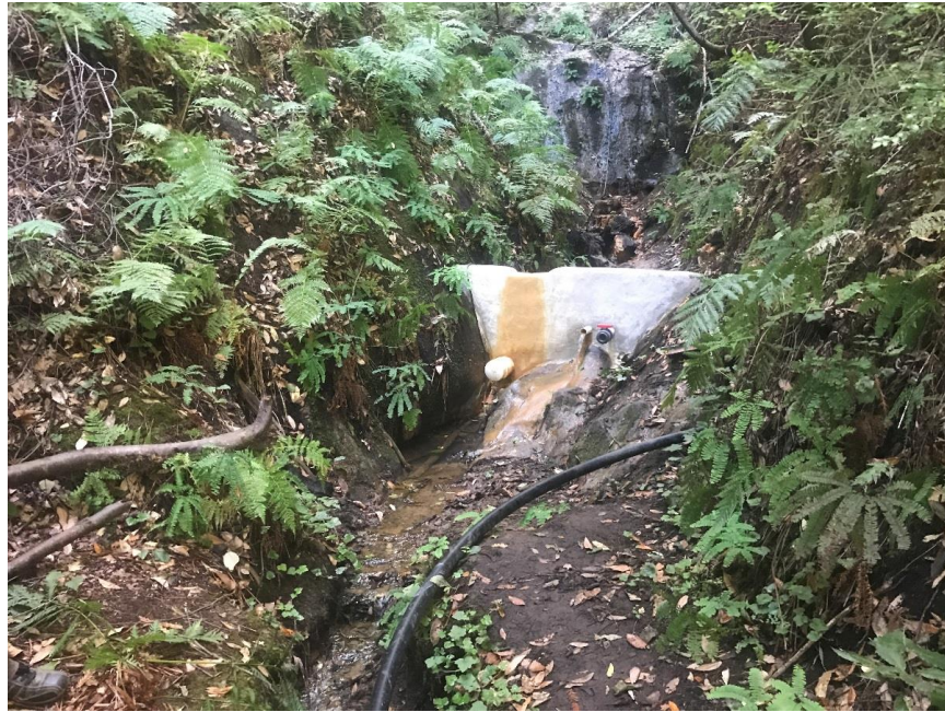
Photo 5. Water Diversion site on Piney Creek.
