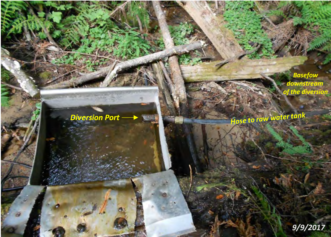
Figure 5. Existing diversion structure on Hoffman Creek, Redwood Glen, San Mateo County, CA. The diversion structure consists of a stainless-steel sink attached to a redwood log across this creek. Sediment and wood debris impounded behind the log has raised the channel bed to allow flow over the log and into the sink. Underflow beneath the log bypasses the diversion, as does overflow when the sink spills.
