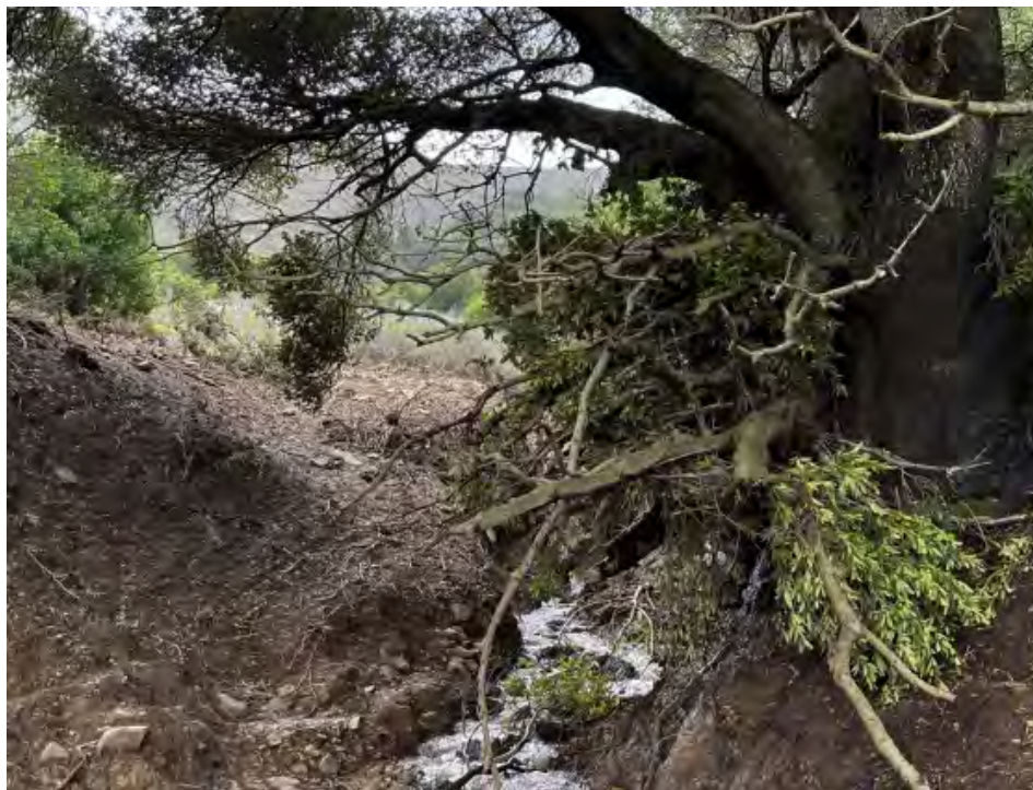
Figure 3. The remainder of the debris dam that likely caused the severe erosion downstream in Owl Canyon. The tree pictured is a California bay laurel, with woody vegetation from other shrubs and trees piled upstream.
