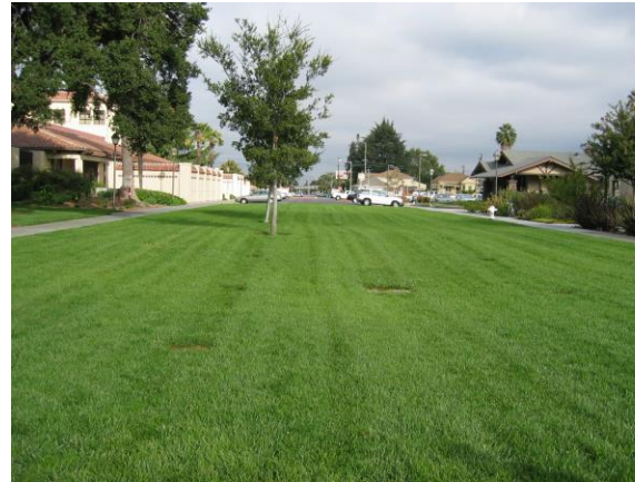
Figure 3-2: Turf block fire access road, Santa Clara University, Santa Clara
