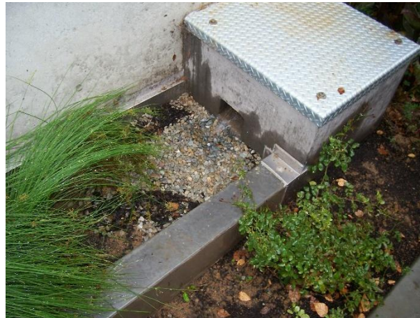
Figure 5-3: Details of flow splitter boxes - Left : Flow splitter vault with weir Right : Flow splitter box with weir (Credit: EOA Inc)
