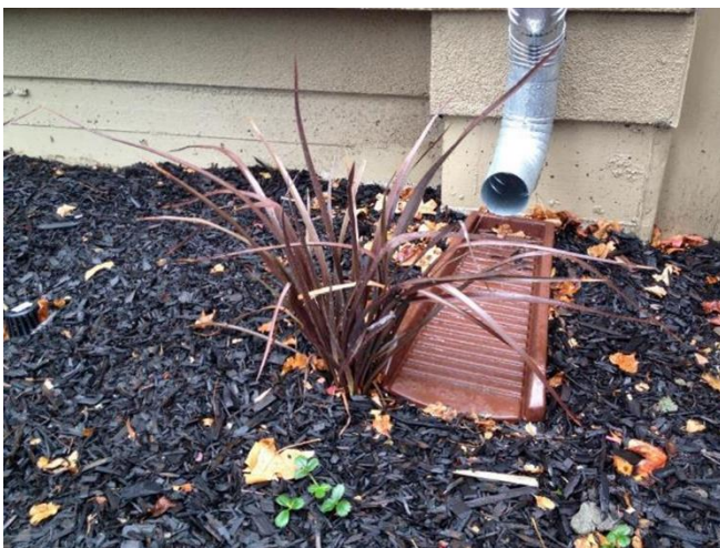
← Figure 5-23: Splash block (Credit: EOA, Inc.)
