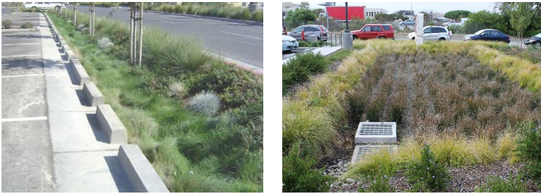
Figure B-2: Examples of Bioretention Areas
