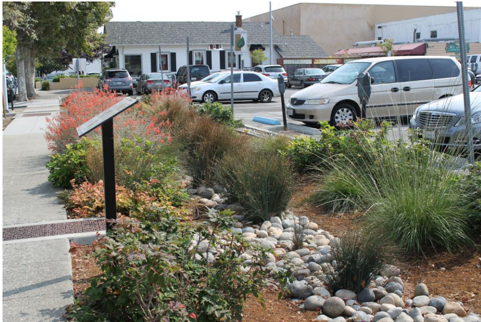
Figure 6-5: Bioretention area featuring several plant types (Credit: City of Burlingame)
