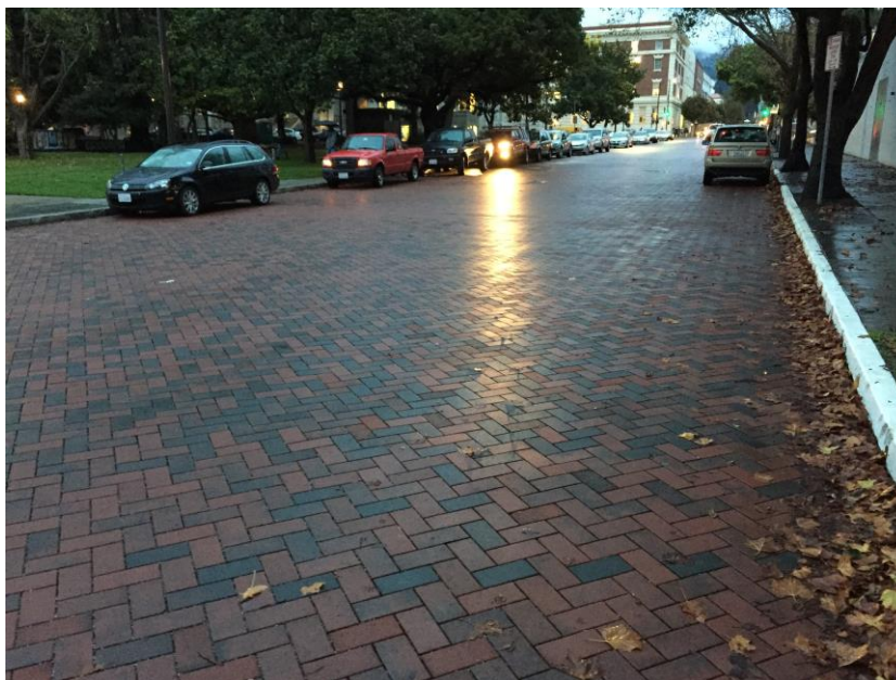
Figure 8-9: Permeable pavers in Berkeley (Credit: EOA Inc.)
