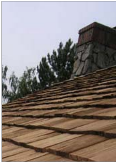
Wood shingle roof Courtesy of Gutter Glove
