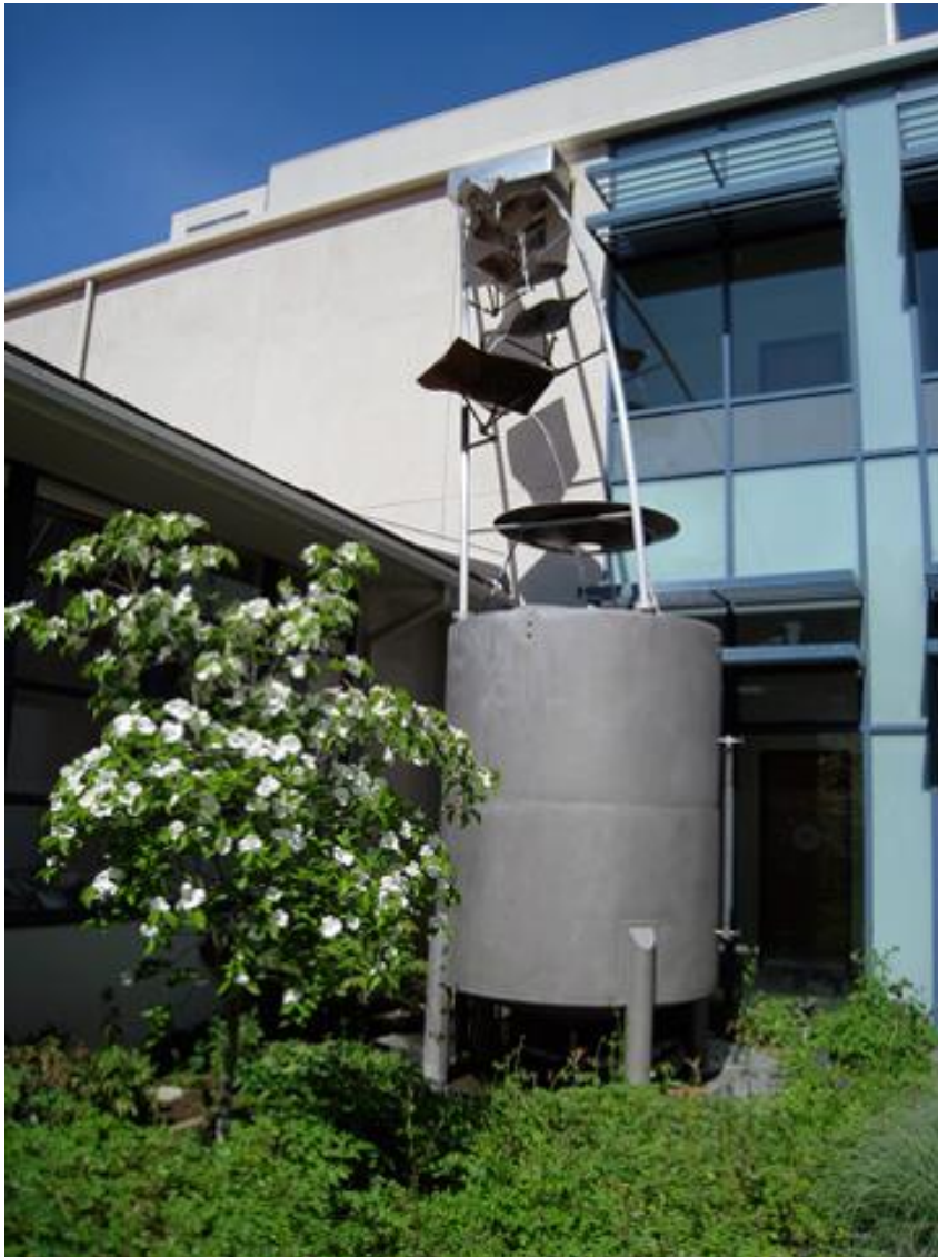
Figure 4-8: Rainwater Harvesting Cistern at Mills College, Oakland (Credit, EOA, Inc.)
