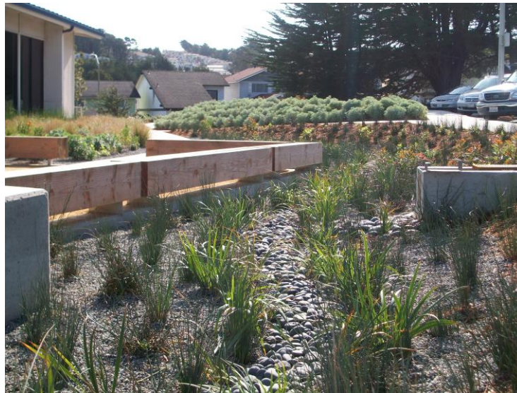
Figure 8-4: Bioretention Area in Daly City (Credit: SMCWPPP)
