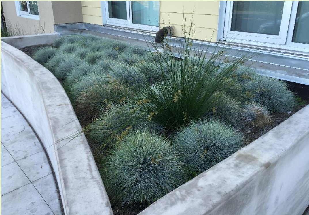
Figure 6-12: Flow-through planter (Credit: EOA, Inc.)
