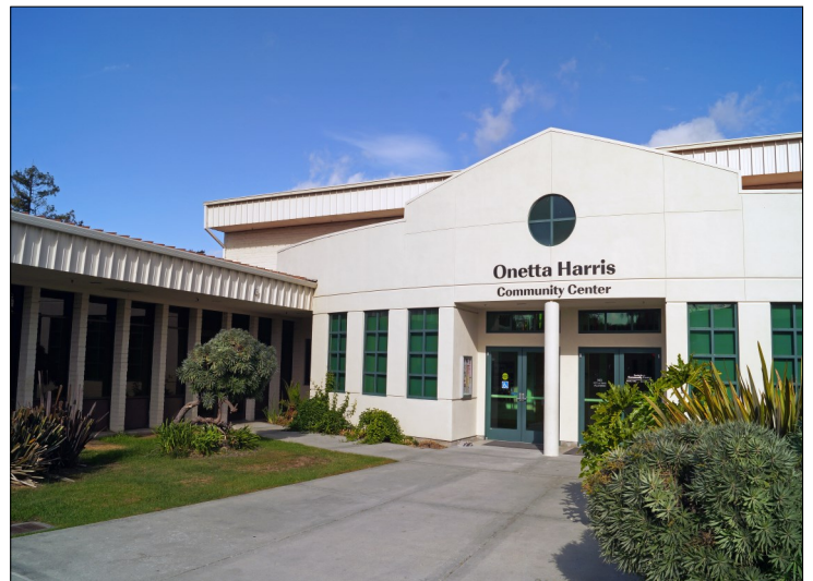
Onetta Harris Community Center, Menlo Park Photo courtesy of County of San Mateo
