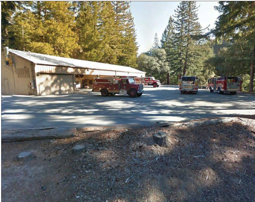
Photograph 19: View of Skylonda Fire Station from Linwood Way across from a residential driveway. Two residences on Linwood Way have direct views of the apparatus building and pavement area.
