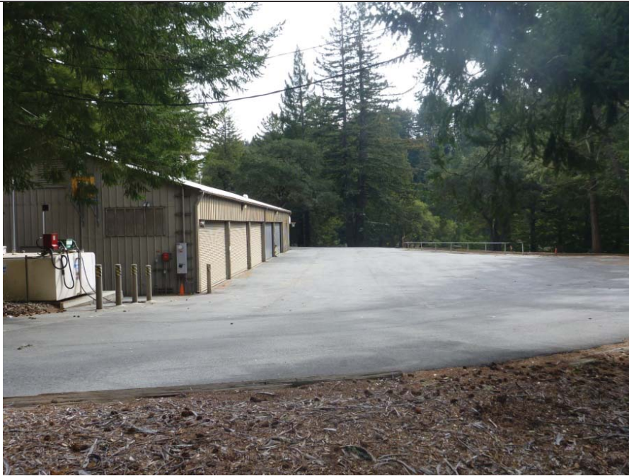
Photograph 9: Apparatus building and paved area from Linwood Way facing south.
