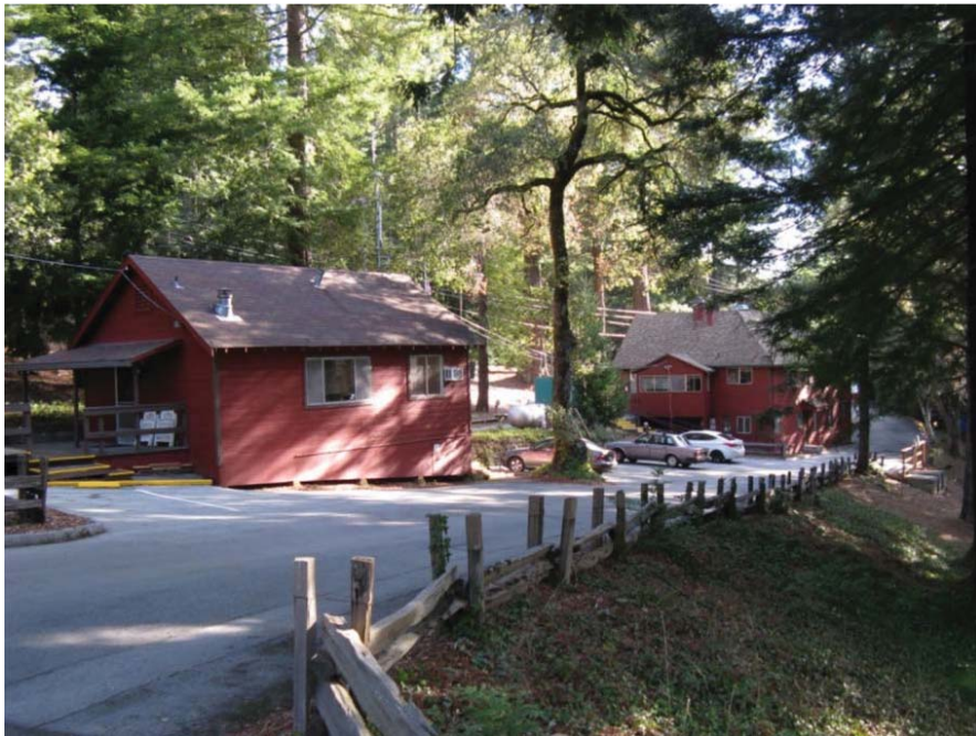
Photograph 8: Administrative buildings from middle of project site. The closer building is the office and the more distant building is the barracks.
