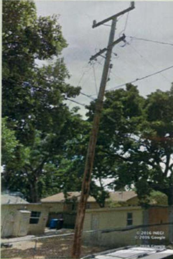
Alternate Pole SOUTH #2- Proposed design does not meet G.O. 95 standards for utility poles
