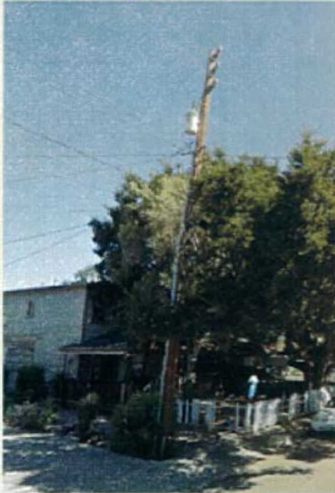
Alternate Pole NORTH #1- Proposed design will not comply with GO 95 regulations
