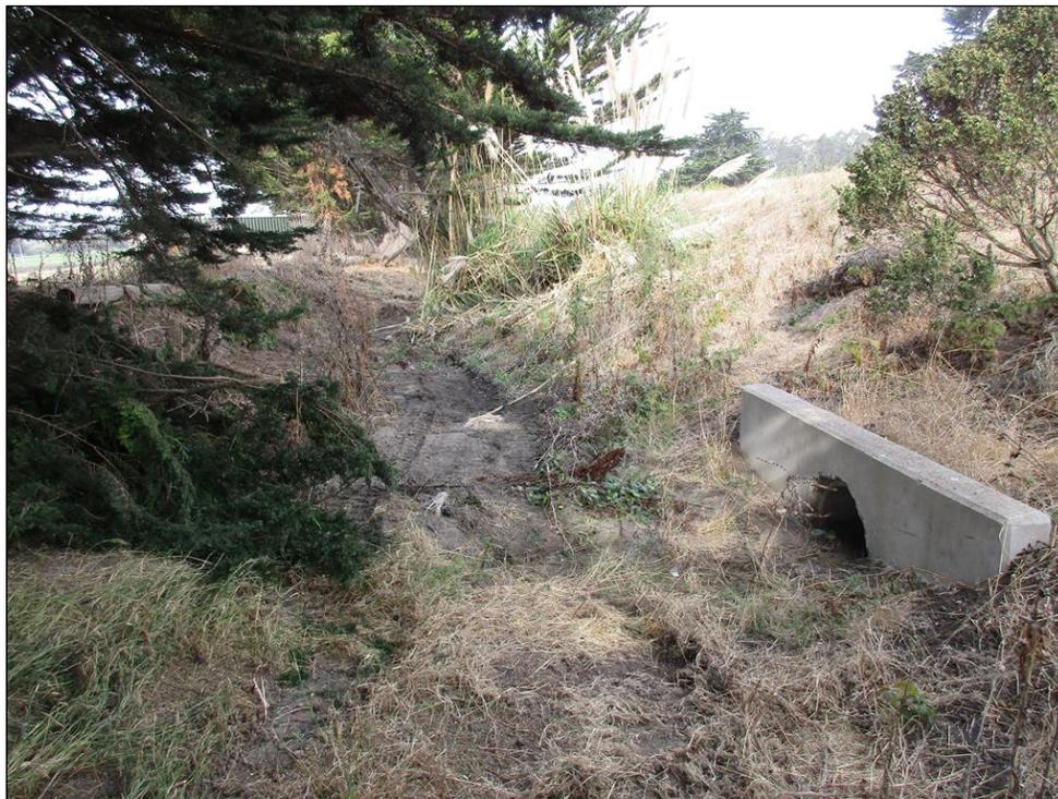
**Photo 4:** View looking northwest along the ephemeral drainage swale along the northeastern boundary of the Project Area. Photo shows the location of the culvert outlet which conveys water from the north side of Cabrillo Highway to the drainage swale.
