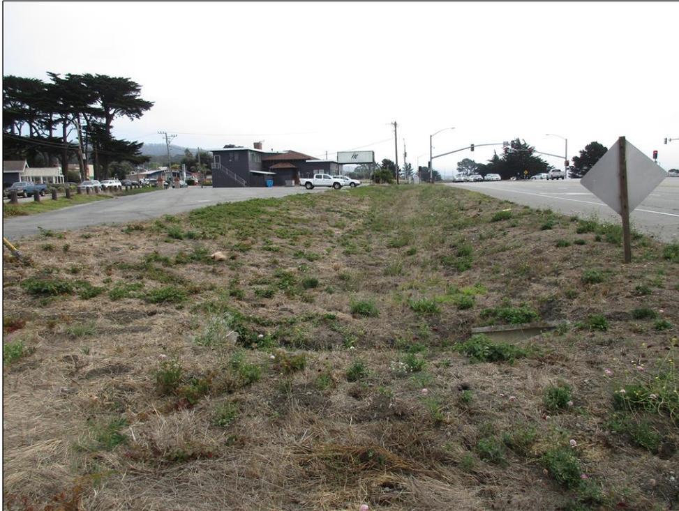
**Photo 5:** View looking south from the northern end of the drainage swale location on the north side of Cabrillo Highway. Photo shows the culvert inlet which conveys water beneath the highway to the drainage swale on the northeastern edge of the Project Area.
